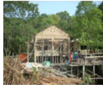
Building the mess house
