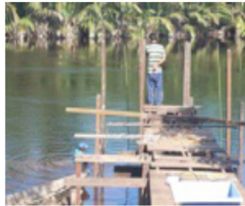
Building the jetty
